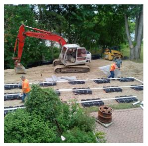
Figure 2. New Tertiary Septic System
