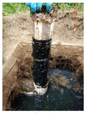
Figure 2. Dirty effluent filter requiring remedial action [Photo credit: Mississippi Rideau Septic System Office]
